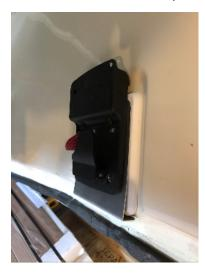
The plate that goes around the latch does not sit nicely and prevents proper closure. Currently this has been removed.
