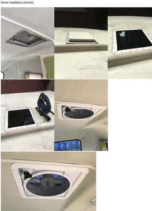
One picture that is missing is the addition of a PVC frame constructed out of 1x2 white PVC planks in order to achieve the thickness required to install the fan.
